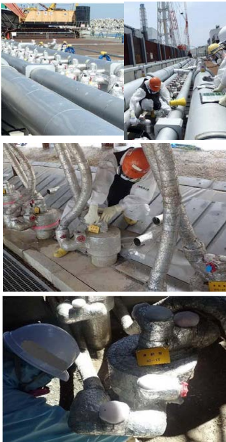
Figure 5: Plaque photos de la mise en route de la congélation (Source Tokyo Electric Power Company Holdings, Inc. Date June 6, 2016).
