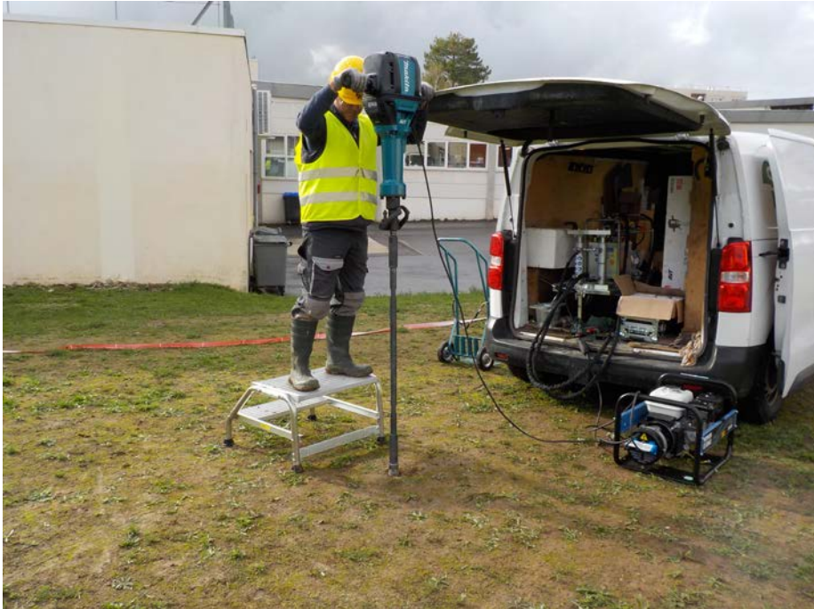
Figure 1 - Intervention au carottier portatif
